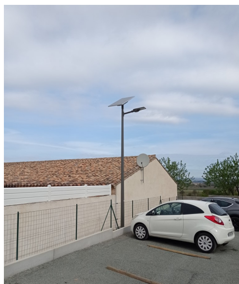
Mur banché Parking des Airettes
